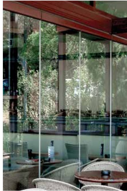
Polycarbonate or PVC weather proofing profiles between the glass, in the whole panel length.
